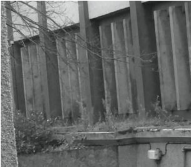
Figure 5.5 Moss on a horizontal surface providing a substrate for vascular plant growth.
